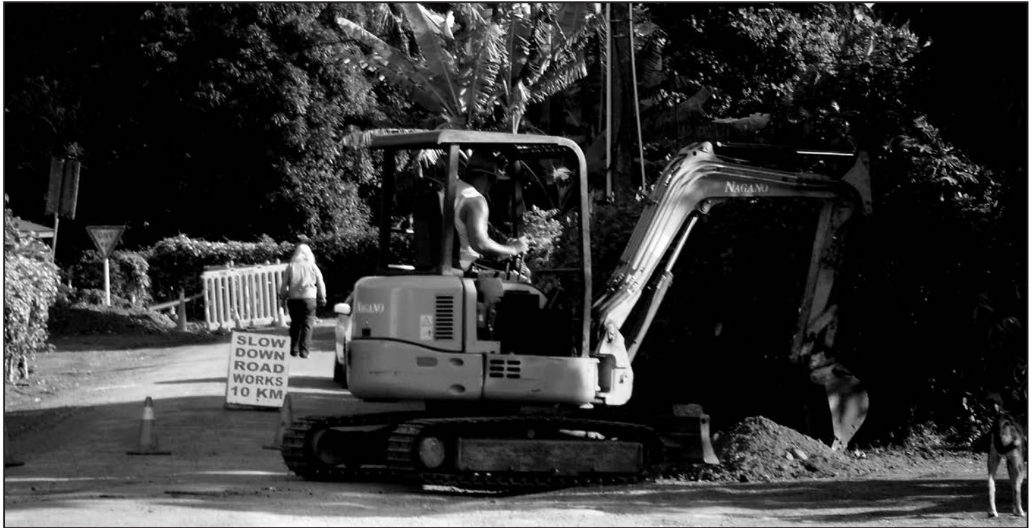
Trenching at Takuvaive Valley road for trunk mains, sub mains and branch mains.
